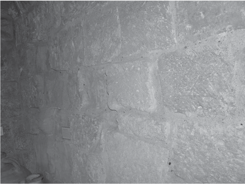
Fig. 36: Limassol Castle, upper level of cells, easternmost cell on south side, right-hand wall showing later masonry skin removed to expose fire-damaged earlier stonework towards the back of the cell [M. Olympios].
